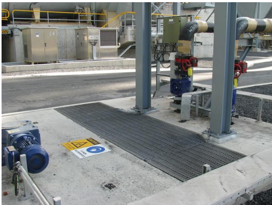
Figure 1 - SCC cooling water pump pit
