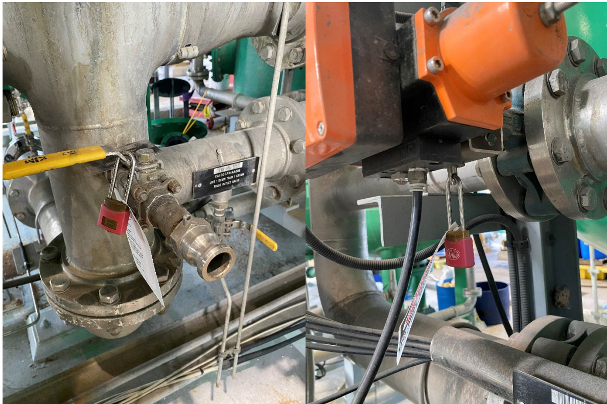
Lockout Device for Blanks / Blinds
